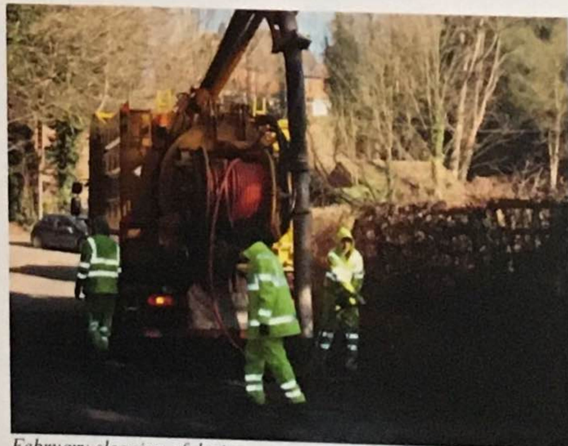
February cleaning of drains
