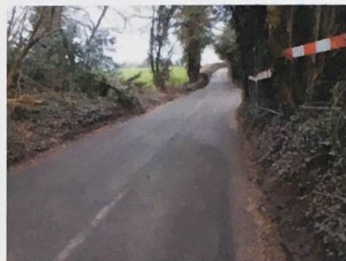
A dry repaired Parrot's Dell
